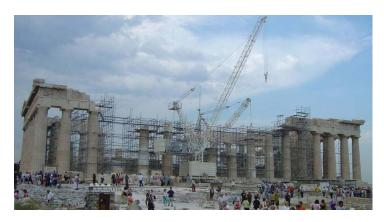
The programme for the North colonnade central zone includes the dismantling and restoration of the entablature and the eight columns that had been restored by Balanos in the 1930s. The rusted metal clamps and dowels are to be removed, new marble is to replace the cement fillings of the previous intervention, and the architectural members, especially the drums, are to be restored to their original positions, in accordance to established methodology. The intervention is scheduled
