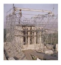
that Balanos had intervened in the past also in 55 blocks of the upper courses of the North wall. As these blocks and courses presented serious problems of structural degradation we had to restore them a new, according to the established methodology (dismantling-structural restoration on the ground-repositioning on the monument).
