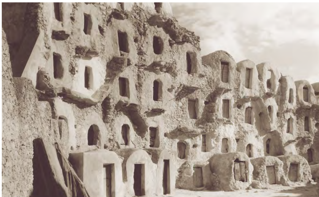
Fig. 97. “Some of the weird stone-plaster-mud constructions, up to five stories high, with outside stairways. Probably chiefly for storage of grain and other products, but part perhaps for dwellings. NOTE: Count de Prorok said these were dwellings. The guide book says storehouses and granaries. The absence of people along the streets bordered by the queer buildings, would seem to carry out the statement of the guide book.” (On verso of one copy, in pencil in an unknown hand: “Strange mud houses at Medenine. Note the outside stairways. Article #3.”) Medenine, Tunisia, April 12, 1925 (Kelsey Museum neg. no. 7.1923).
