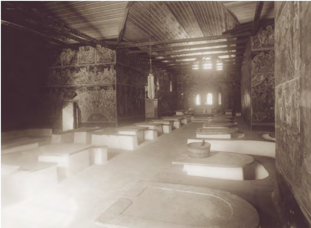
Fig. 105. View down the long axis of the refectory showing drainage arrangements and walls covered with mural paintings, Lavra Monastery, Mount Athos, Greece, July 4–6, 1925 (Kelsey Museum neg. no. 8.0211).
