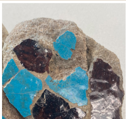
Left: Details of treatment for the glazed stucco. In the upper image, the white putty Laurel applied is visible; in the bottom photo, the adhesive has been painted over.
