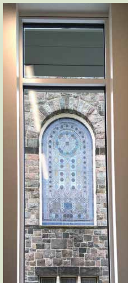
The Kelsey's Tiffany window from the south stairwell in the Trotter Center. Photo by Dawn Johnson.
