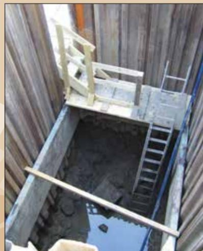
A view of the deep trench from above as the pump (slender blue tube just right of ladder) is working to drain the water.
