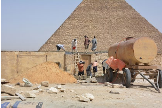
Figures 4–5. Repairing the roof of the laboratory, which had been damaged by heavy rains. Photos by Richard Redding.
