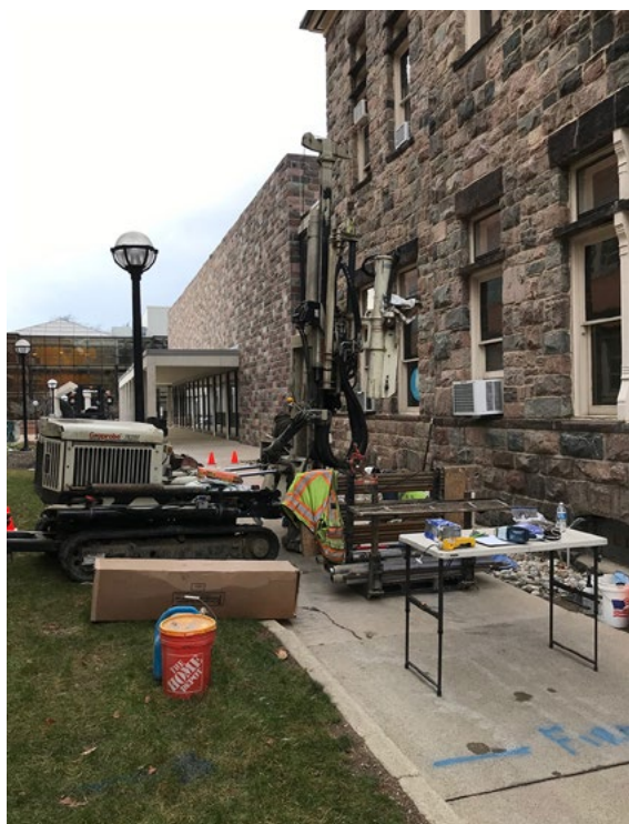
Figure 4. Mannik & Smith boring soil on the south side of the Kelsey Museum. Photos by Dawn Johnson.
