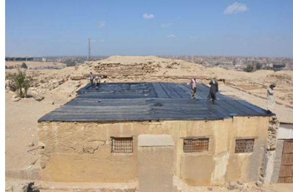
Figures 4–5. Repairing the roof of the laboratory, which had been damaged by heavy rains. Photos by Richard Redding.
