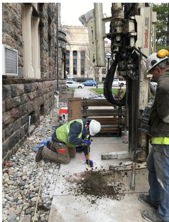
Figure 4. Mannik & Smith boring soil on the south side of the Kelsey Museum. Photos by Dawn Johnson.
