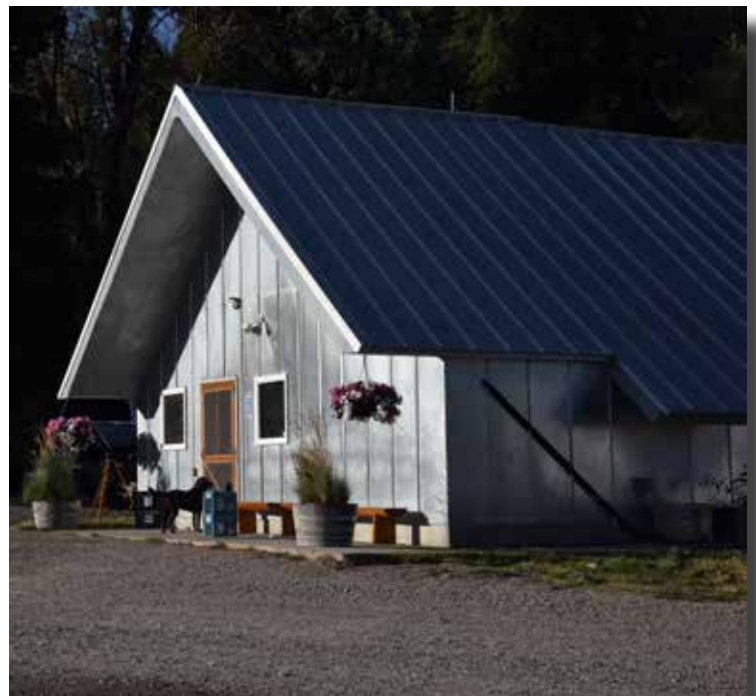
The Camp Davis Mess Hall is one of the oldest buildings at Camp Davis, dating back almost 90 years. An addition to the Mess Hall that includes both a walk-in cooler and freezer was added in 1990, with the help of a generous gift by Drew Issacs and Jan Kappmeyer. The importance of a functioning dining hall to Camp Davis classes, along with changing health and building codes, brings us to a point where we need to explore options for a Mess Hall renovation in the near future. Planning efforts will take place over the next few years to determine the scope and cost of renovating the Mess Hall. Photo by Kacey Lohmann
