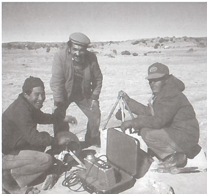
Figure 2. Geophysicists at a borehole site, making temperature measurements with an electrical resistance thermometer.
