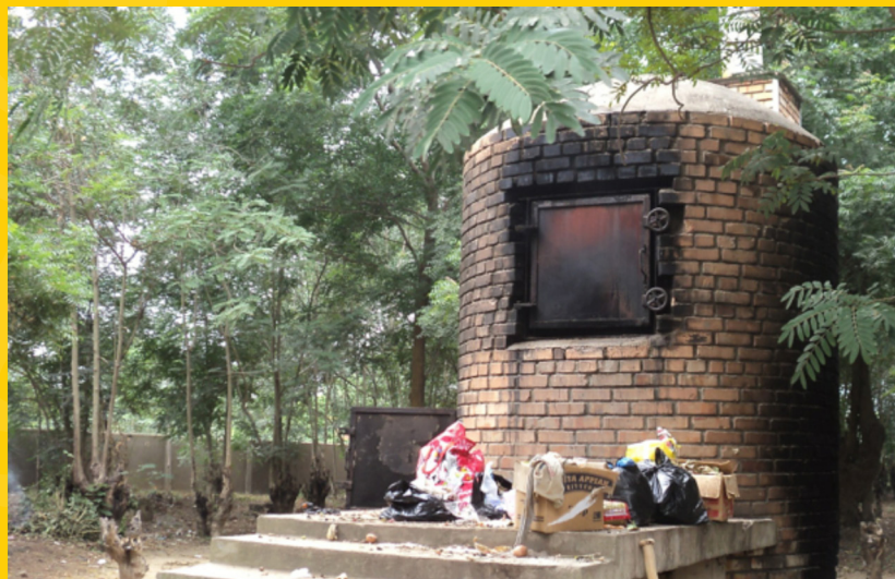
On-site incinerator at a public hospital in Ghana: problem or solution for medical waste? Courtesy of Emilia Udofoia.
