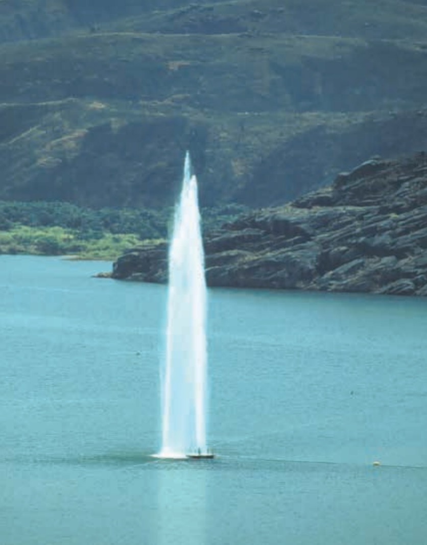
Once started, the degassing fountain at Lake Nyos is self-sustaining
