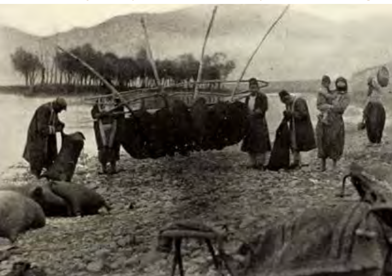
Armenians Constructing a Raft of Inflated Sheepskins on the Banks of the Euphrates River. Photo by Ellsworth Huntington
