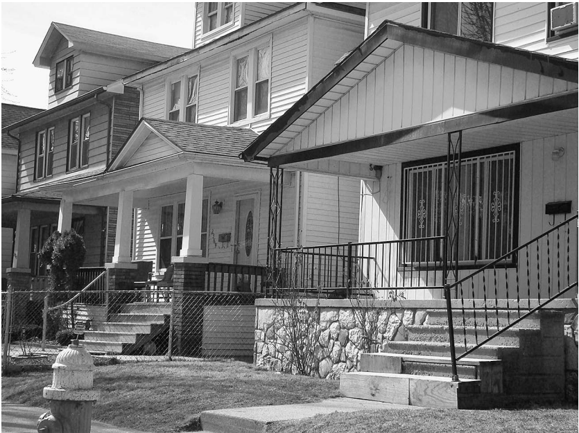
Figure 9. Window treatments that enhance eyes on the street. Photograph by author.
