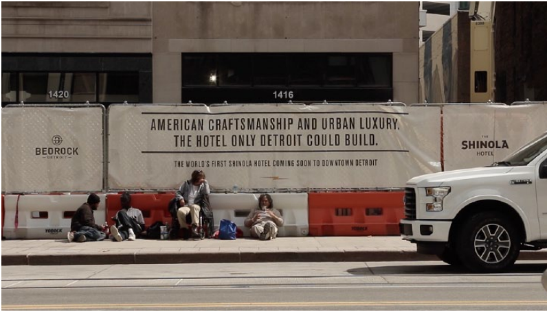
Figure 1. A group of Detroiters sit on a Downtown sidewalk in front of a construction site for a new luxury hotel built by the Shinola leather company. A few minutes after this photo was taken, this area was cleared by private security and Detroit police. Photo © Philip Conklin.
