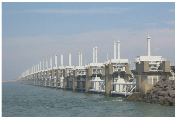
Storm Surge Barriers
